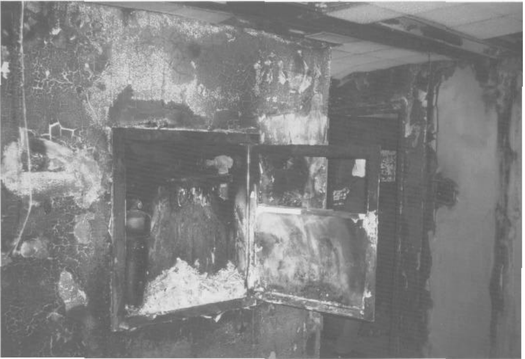
Occupant use standpipe hose cabinet on 26th floor.
