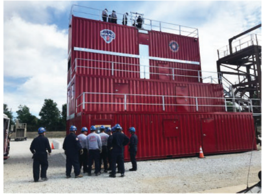
MAAC’s burn tower part of the extensive training facilities
